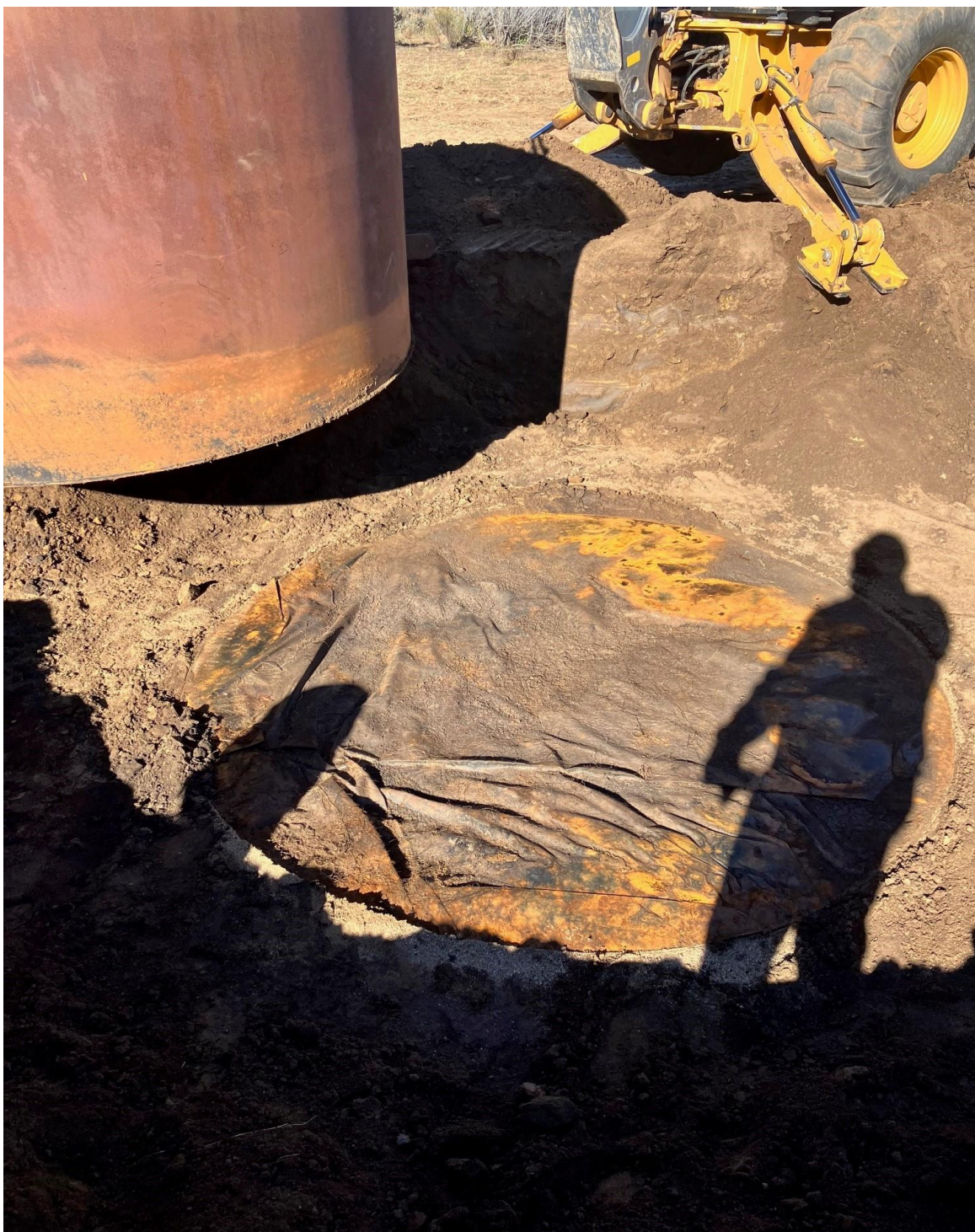
Photo 2: BGT Being Removed with Liner in Bottom of Cellar
