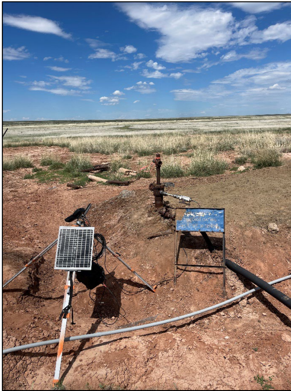
3) TLSA #005 (30-005-60572) - Methane Flow Test Rig Up
