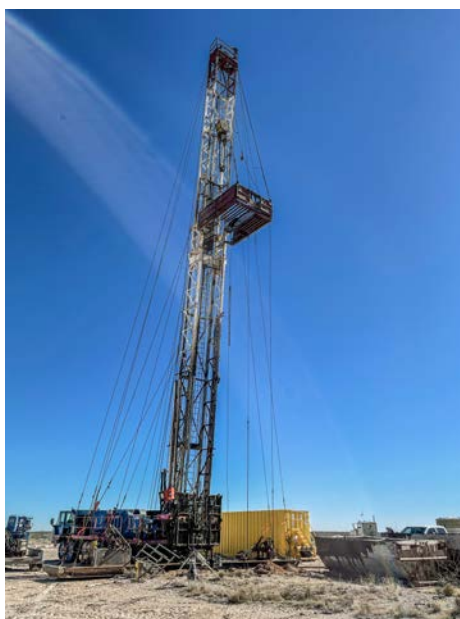
Shelly State #006 Plugging
