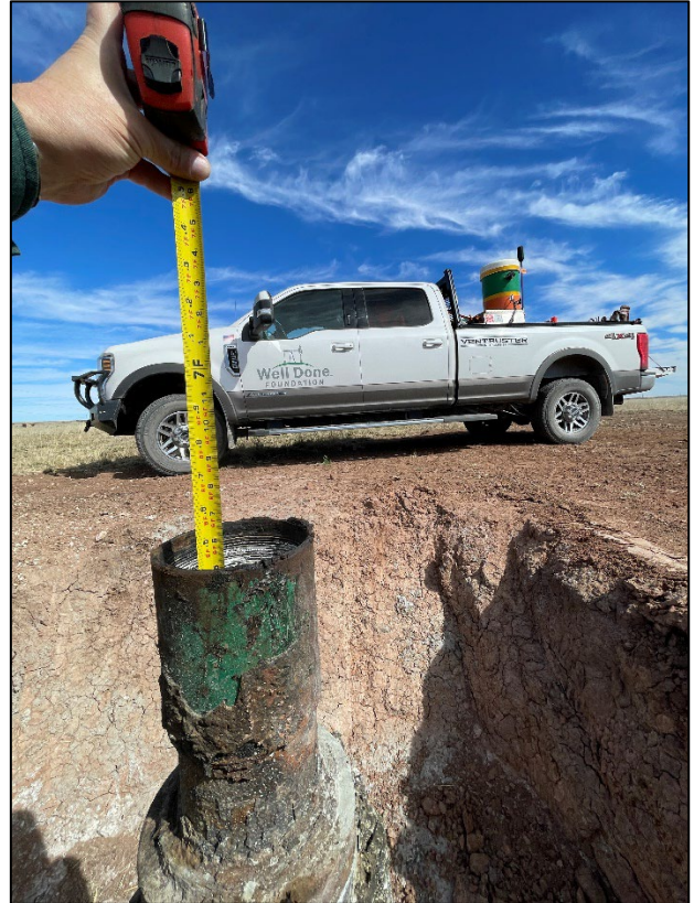
2) O'Brien Fee 25 #005 – Post Plug Cement filled to within -6'-5"
