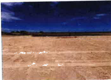
View to W of excavation (5/17/23).
