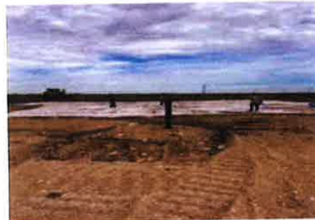
View to W of bentonite in pit area (5/18/23).
