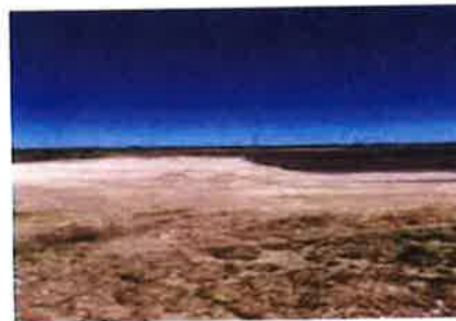
View to N of backfilled excavation (6/14/23).
