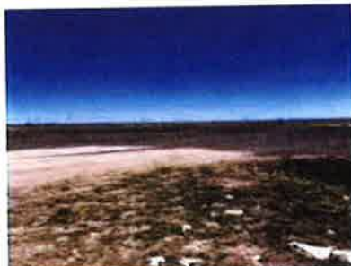
View to W of backfilled excavation (6/14/23).
