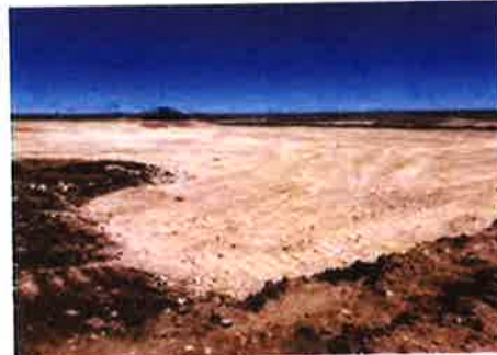
View to NW of excavation (5/8/23).
