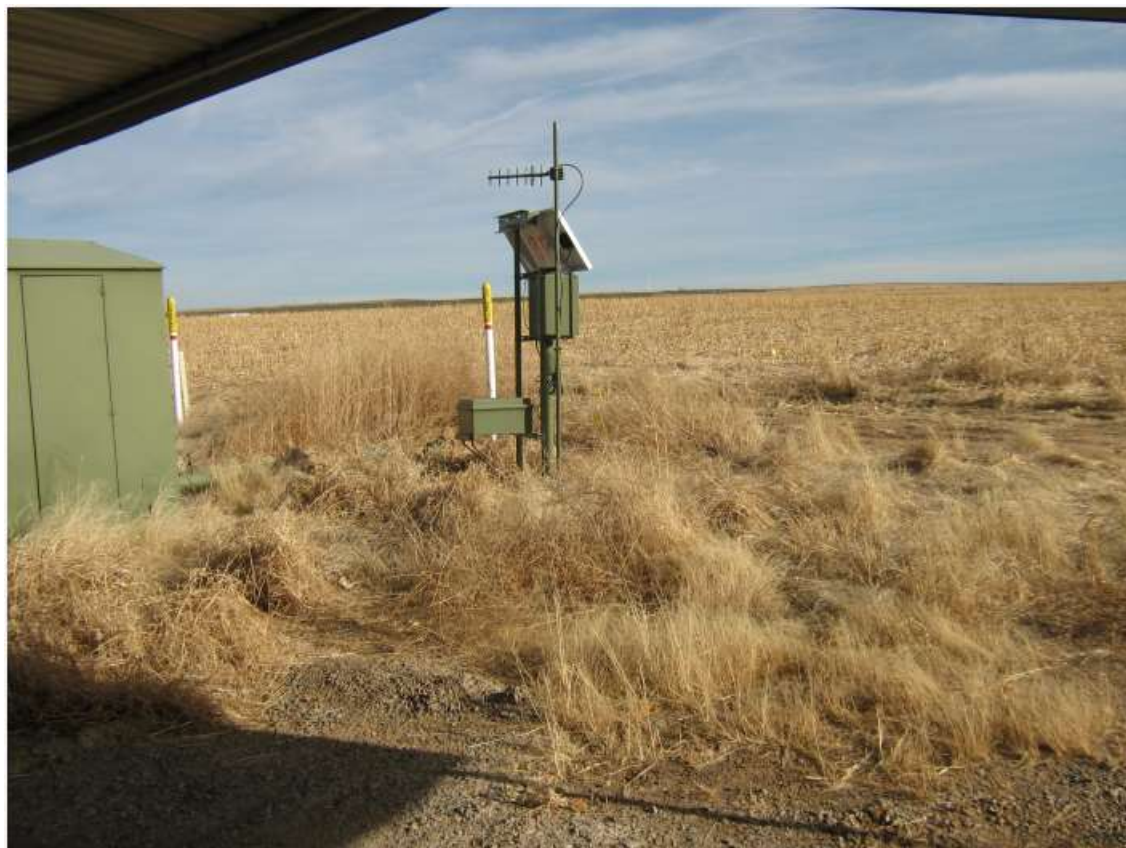
Meter Run with RTU, Solar Panel and Batteries
