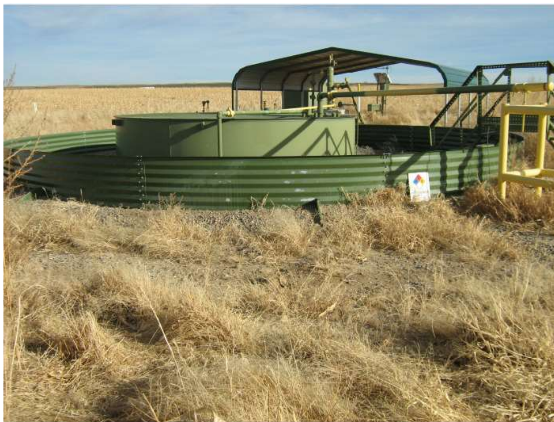
Photo of pit tank – above grade LPT with metal containment ring Serial #30697-72 (95 BBL)
