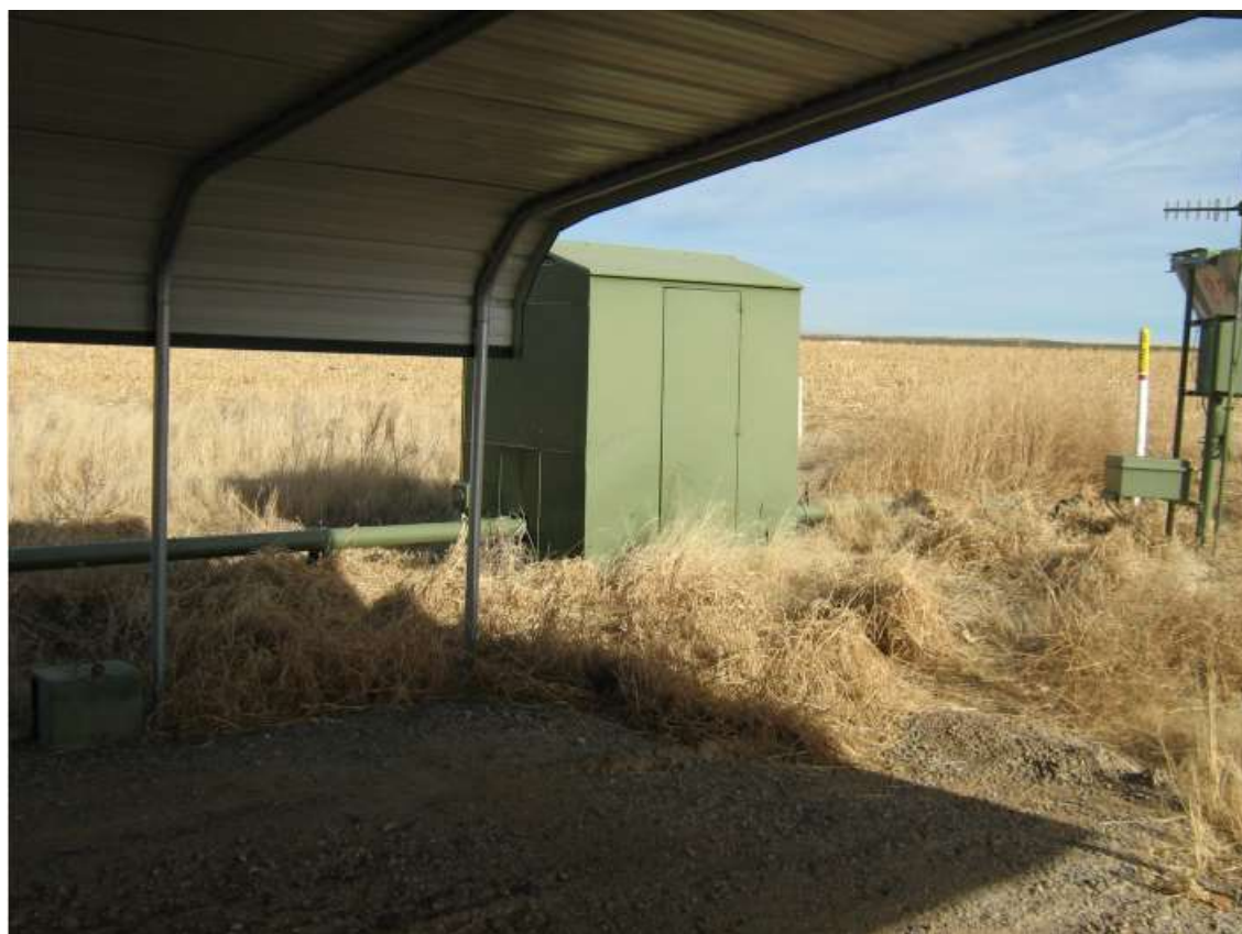
Meter House with 4 inch meter run #97883
