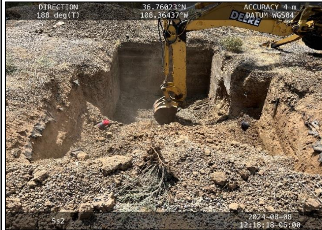
Photograph: 6 Date: 8/8/2024 Description: Initial potholing activities View: South
