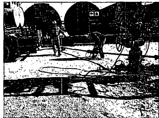
Image 5: Petroplex employees laying pipe from pump truck to well head.
