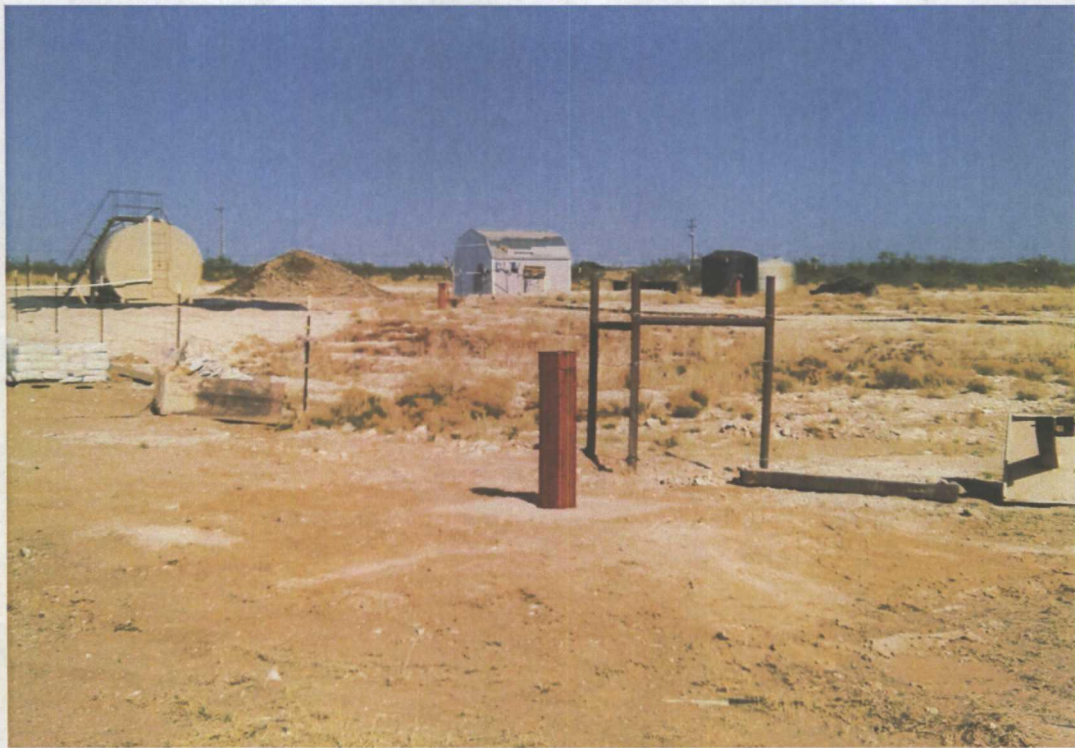
MW-7A above ground vault
