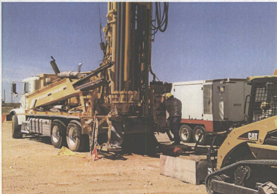
Rigging up on MW-8A
