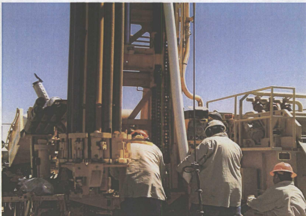
Installing casing in MW-2A
