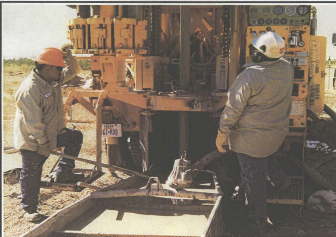
Drilling MW-2A with mud
