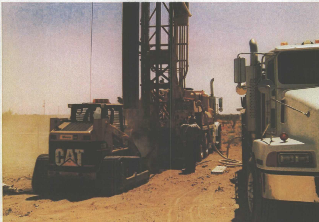
Drilling MW-7A with air
