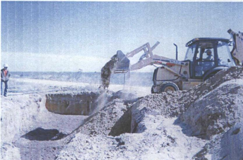
Backfilling site above clay liner
