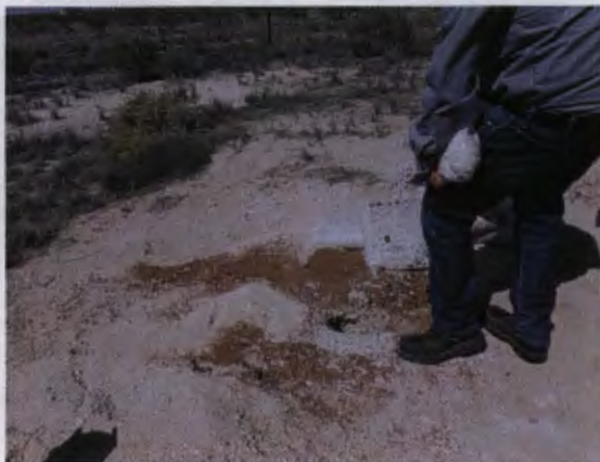
Plugging SB-1 in total with bentonite, 6/21/13
