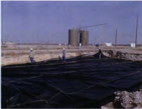
Installing the 20-mil, reinforced liner at approximately 4.5 ft bgs, facing northwest
