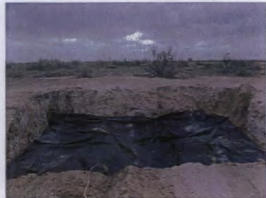
Installing 30'x30' 20 mil plastic liner @ 6' bgs 10/12/2012
