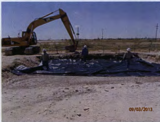
Installing liner, facing south 9/3/2013
