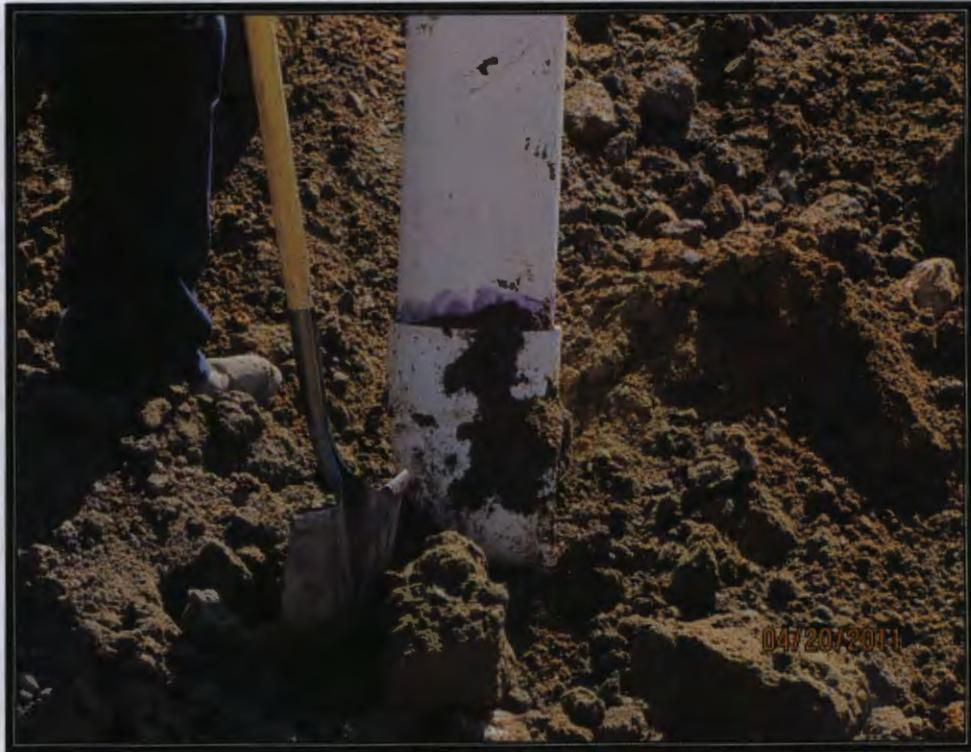
Photo 5: Bottom of Leak Detection System, No Concrete Found
