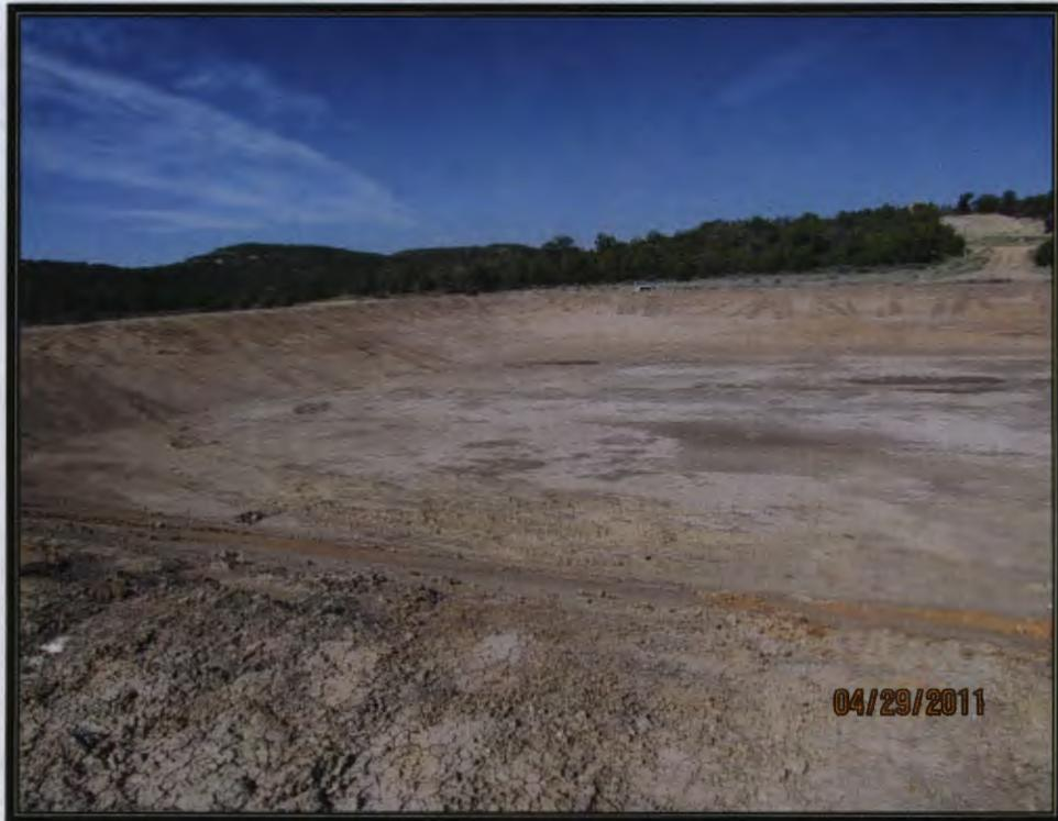
Photo 7: Pond after Liner and Leak Detection Removed
