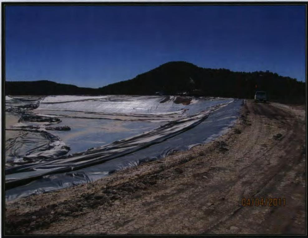
Photo 2: Removing the Liner
