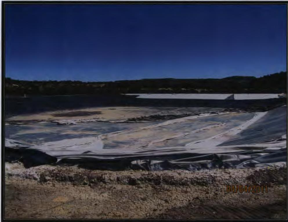
Photo 3: Removing the Liner
