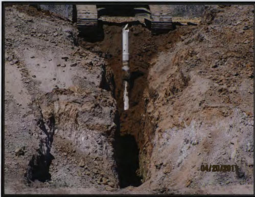
Photo 4: Removing the Leak Detection System
