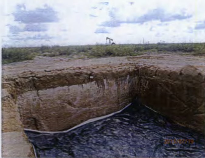
Installed 30' x 30', 20 mil reinforced poly, facing southeast 7.19.13
