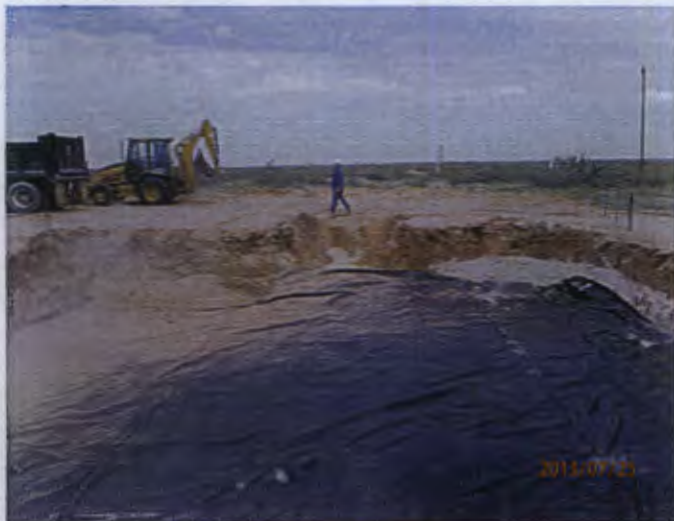
Padding above 2 nd 20 mil reinforced Liner, facing North 7.25.13
