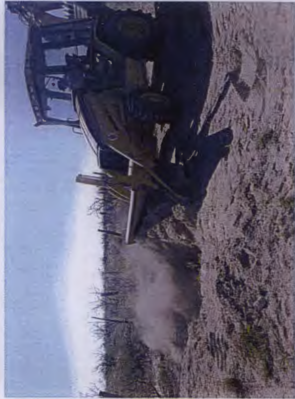
Backfilling excavation
