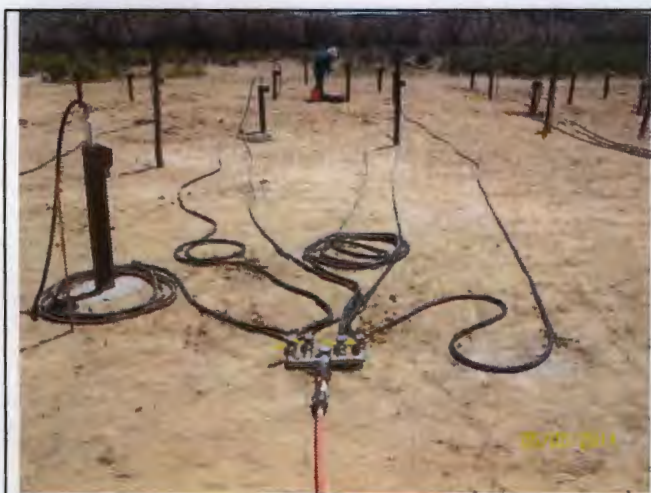
3.) Injection points connected via manifold to the pumping trailer.
