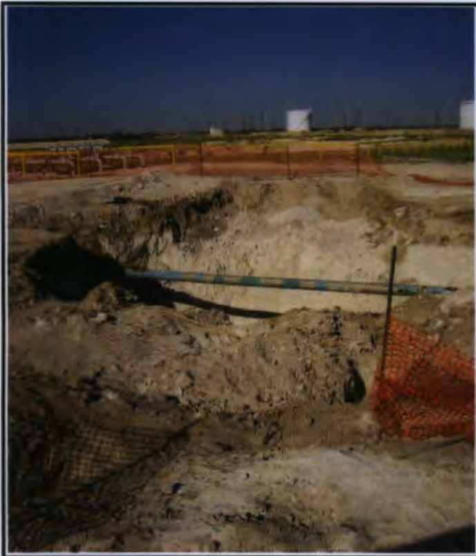
1.) Representative view of the leak source, immediately after discovery of the release.
