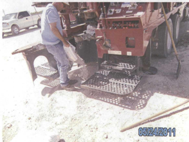
Plugging SB-4 in total with bentonite
