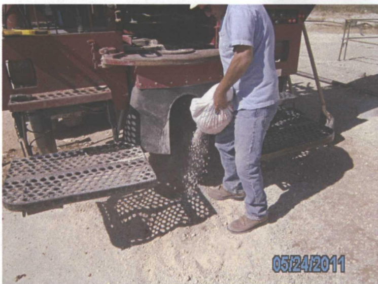
Plugging SB-3 in total with bentonite
