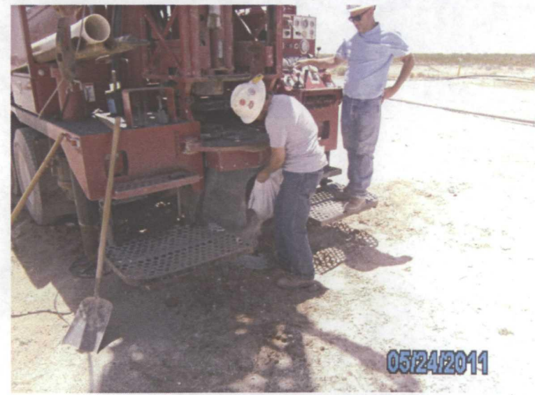
Plugging SB-6 in total with bentonite 5/24/2011
