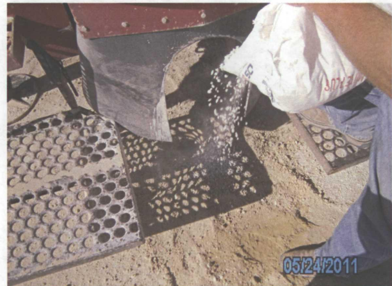
Plugging SB-2 in total with bentonite
