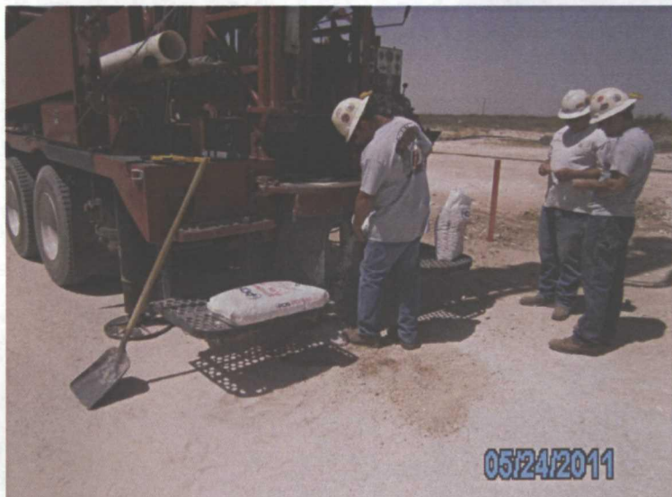
Plugging SB-5 in total with bentonite 5/24/2011
