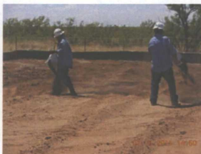
adding restorNance to the backfilled site, facing northwest 7/15/2011
