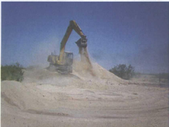
blending the excavated soil, facing west 6/10/2011
