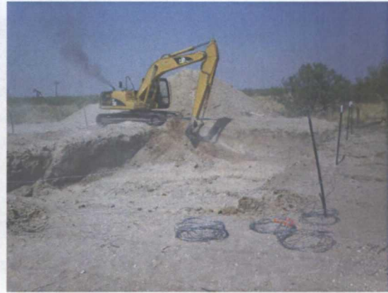
excavating the north side of the site to a depth of 7 ft bgs, facing southwest 6/8/2011
