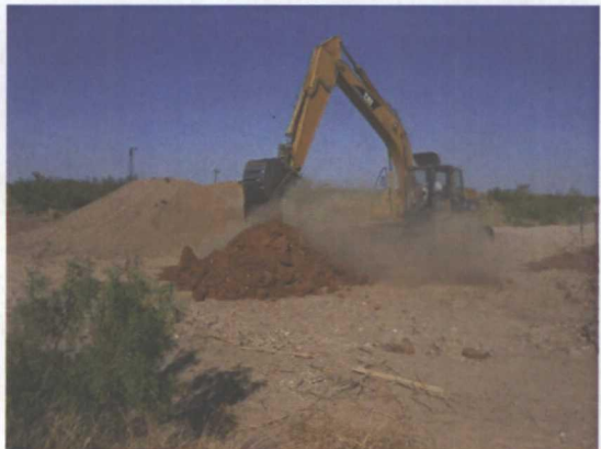
blending excavated soil with imported soil, facing southwest 6/25/2011
