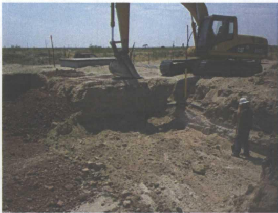
completed excavation with the existing clay barrier located, facing east 6/9/2011
