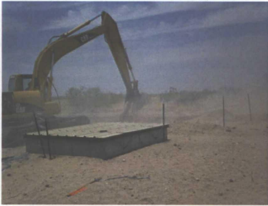
backfilling the north side of the excavation with blended backfill, facing northwest 6/13/2011
