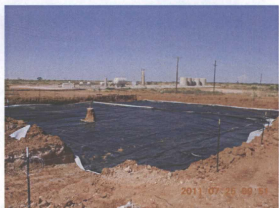
Liner installed, facing southwest 7/25/11
