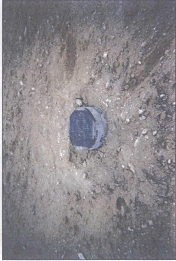
ID Plate Marking Liner at Backfilled Site
