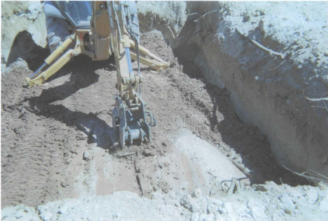
Figure 4 – Compaction of installed clay infiltration barrier upon removal of former junction box.
