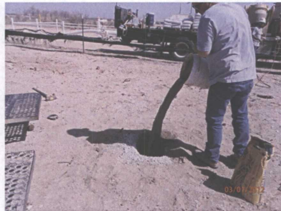
Plugging the well with a 1-3% bentonite/concrete slurry
