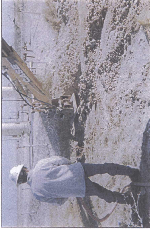
backfilling and compacting 12/2/2005
