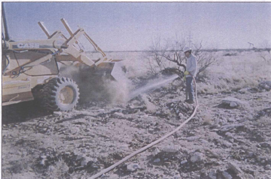
backfilling and compacting trench
