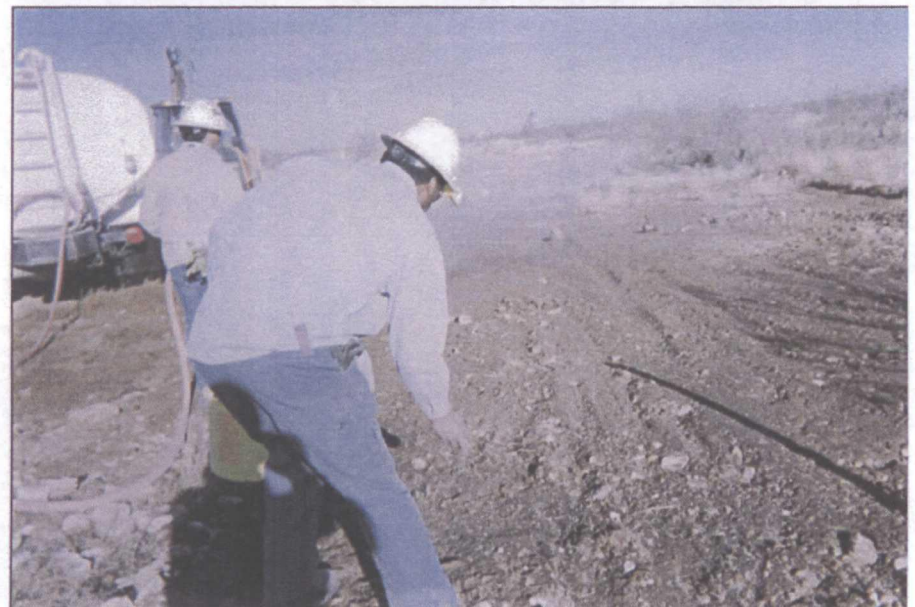
seeding and watering backfilled site
