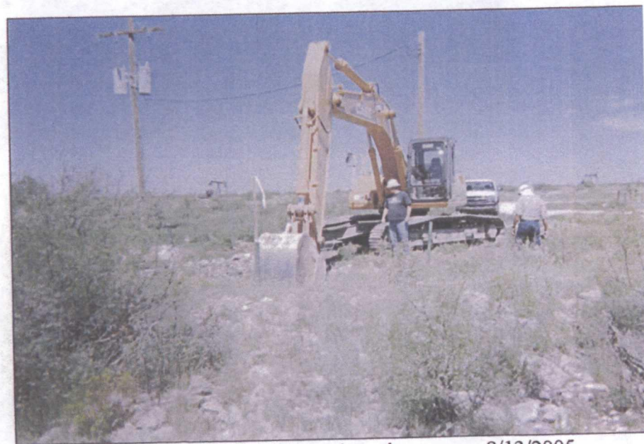
delineation trench at former box site
