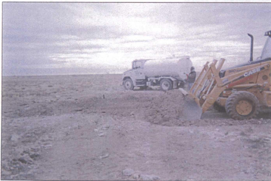
spreading imported topsoil on backfilled site
