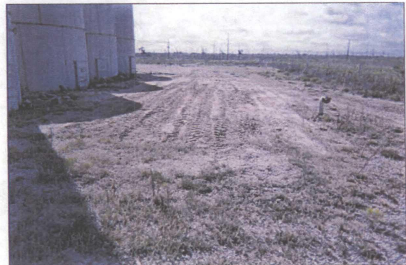
site backfilled with 12 yds 3 imported fill
