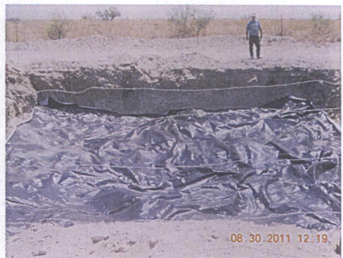
Installing a 30x30-ft., 20-mil reinforced liner at 5-ft. BGS, facing east 8.30.11
