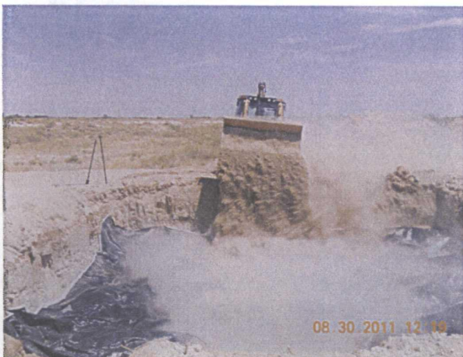
Backfilling site above liner, facing north 8.30.11
