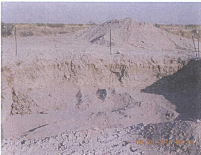
Excavation prior to installation of plastic liner up to 5-ft. BGS, facing west 8.30.11
