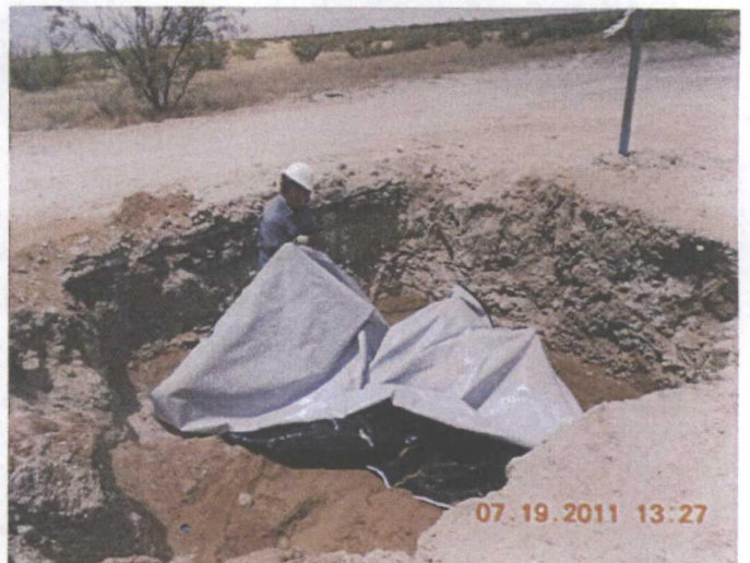
Installing liner, facing northwest
