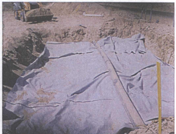
Installing a 30x20-ft., 20-mil reinforced liner at 4-ft. BGS, facing north 5.2.11
