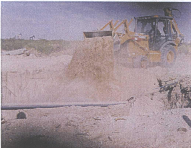
Backfilling the excavation up to 4-ft. BGS, facing west 5.2.11
