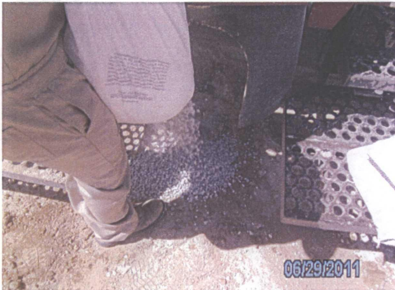
Plugging SB-1 with bentonite, facing north
