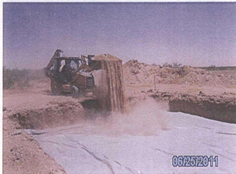
Backfilling above installed plastic liner, facing north
