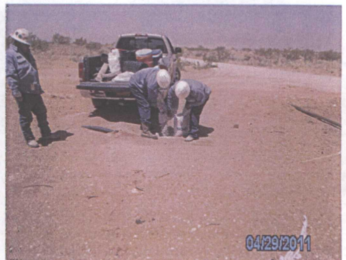
Plugging SB-1 with bentonite, facing west
