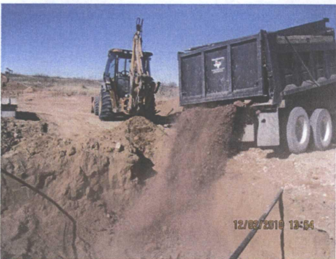
Importing clay for liner, facing north 12.2.10
