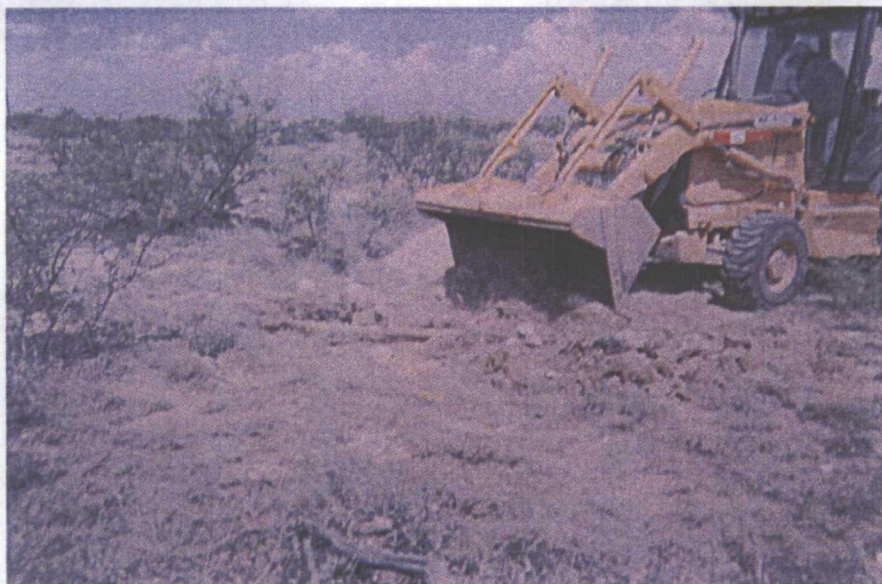
Backfilling excavation
