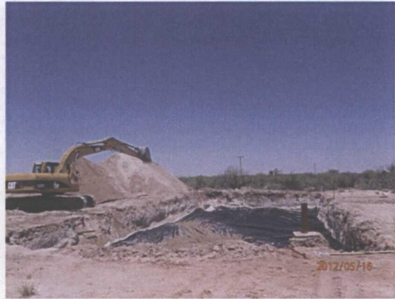
Backfilling above installed 39' x 81' 20-mil reinforced plastic liner, facing north 5/16/2012
