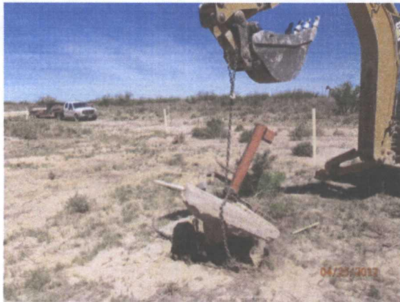
Pulling MW-1, facing northwest 4/25/12
