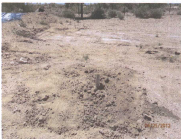
Plug and abandon MW-3 completed 4/25/12
