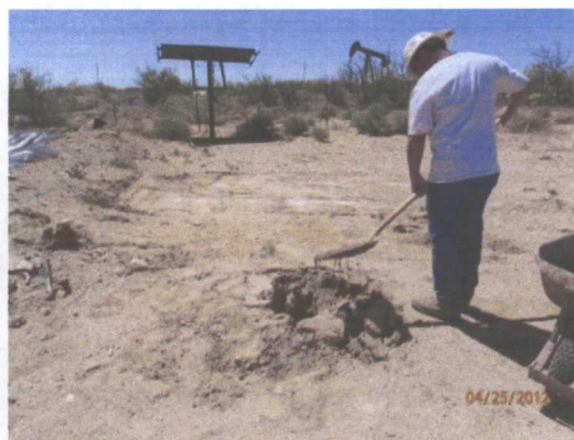
Plugging MW-3 with 1-3% bentonite/concrete slurry and 3 ft concrete cap 4/25/12
