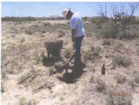
Plugging MW-2 with 1-3% bentonite/concrete slurry and 3 ft concrete cap 4/25/12
