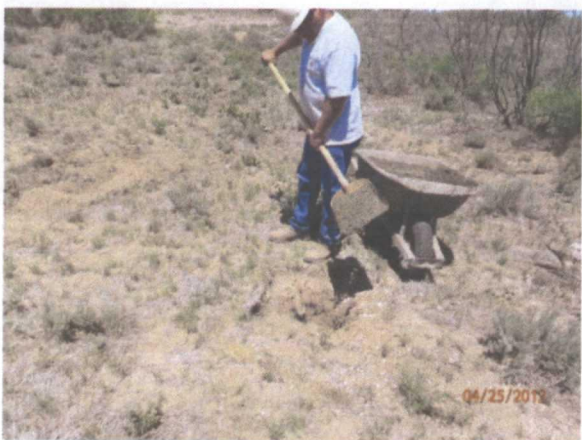
Plugging MW-4 with 1-3% bentonite/concrete slurry and 3 ft concrete cap 4/25/12
