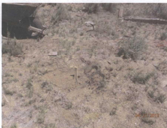
Plug and abandon MW-4 completed 4/25/12
