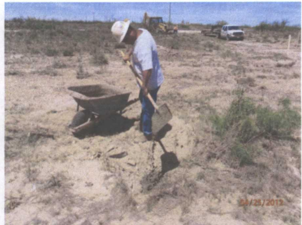
Plugging MW-1 with 1-3% bentonite/concrete slurry and 3 ft concrete cap 4/25/12
