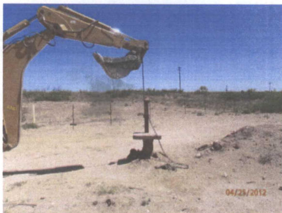
Pulling MW-3, facing northeast 4/25/12
