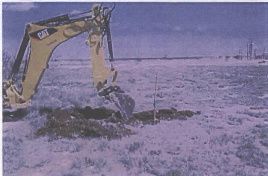
Delineation trench being excavated
