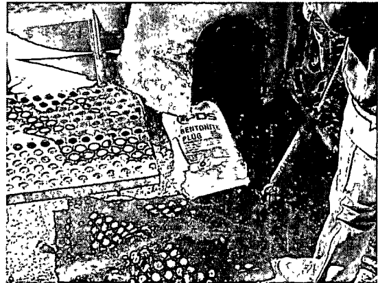
Completed temporary monitor well
