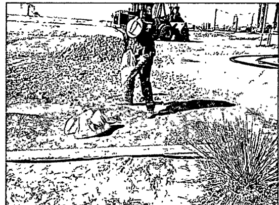
Plugging the well in total with bentonite, facing east 5/11/11
