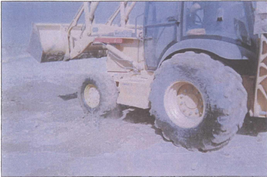
completing backfill; spreading topsoil 2/16/06
