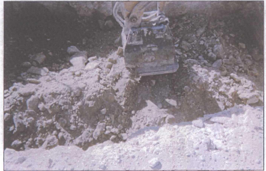
compacting backfill 2/15/06
