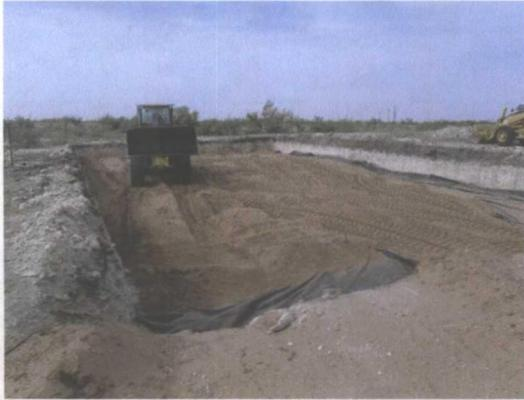
Installing 1' sand lift above liner, facing south
