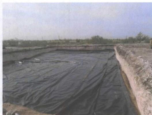
Installed 48' x 96', 20-mil reinforced plastic
