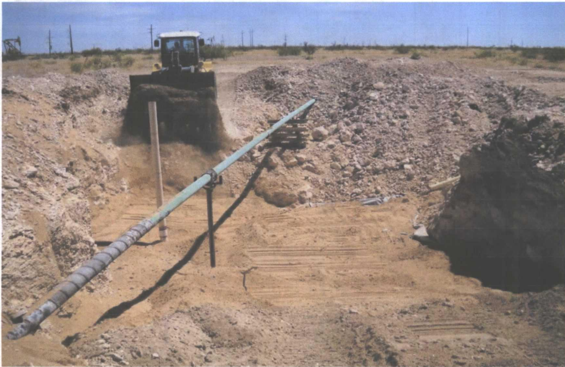
Chevron Grayburg 6-Inch Sec. 6 (Historical) - Installation of Pad Sand
