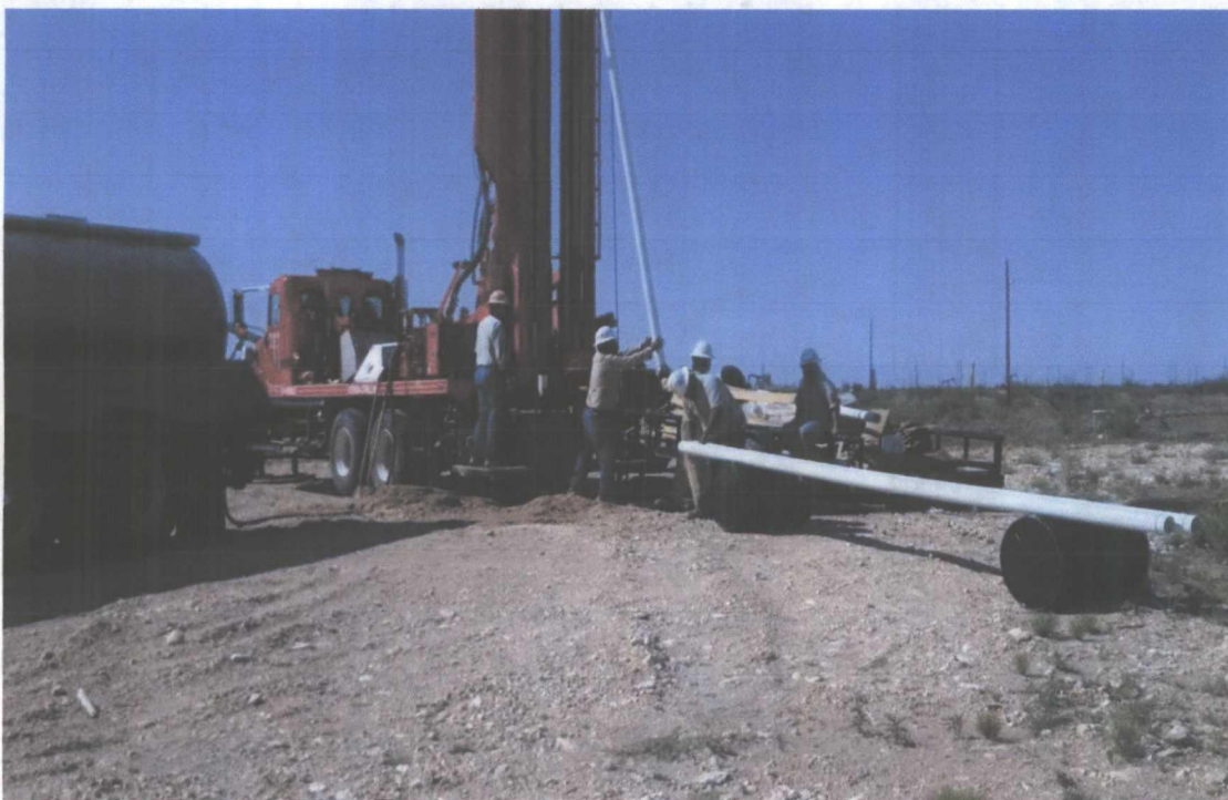
Chevron Grayburg 6-Inch Sec. 6 (Historical) - Installation of 4-Inch PVC Riser in Monitor Well MW-4
