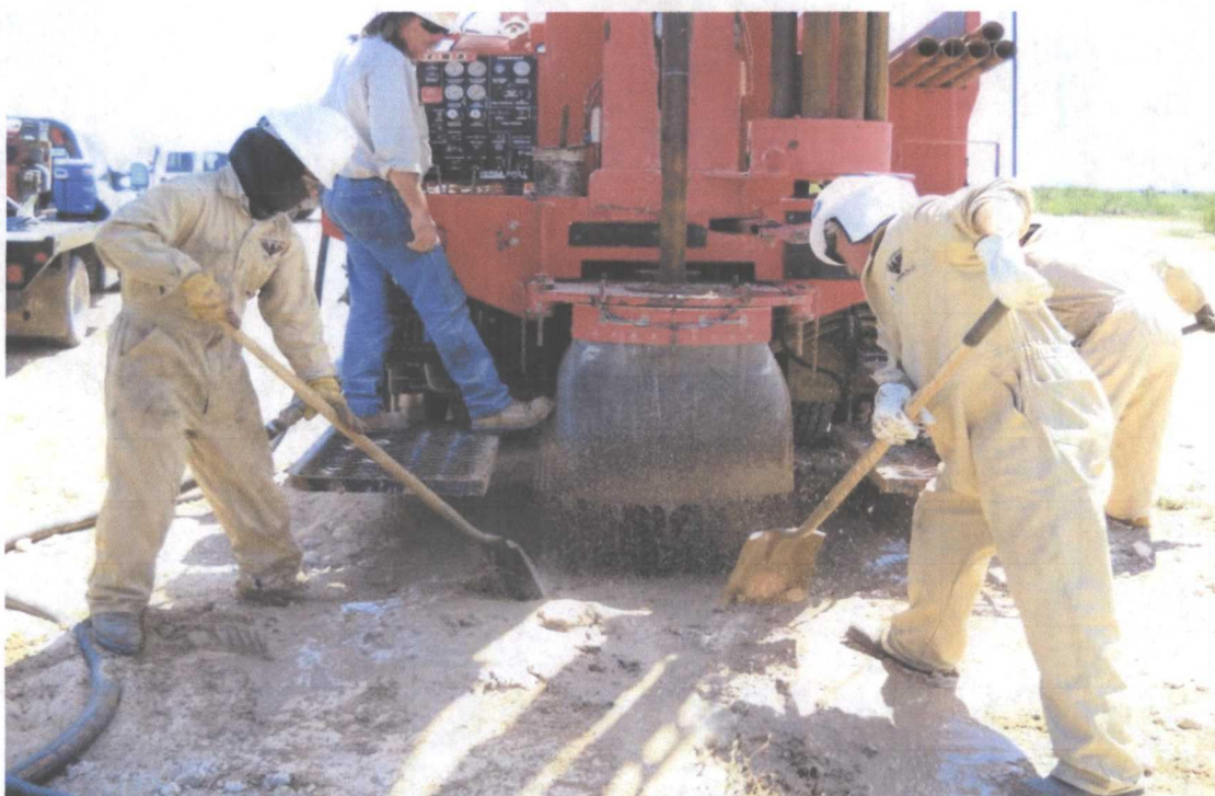
Chevron Grayburg 6-Inch Sec. 6 (Historical) - Advancement of Monitor Well MW-1
