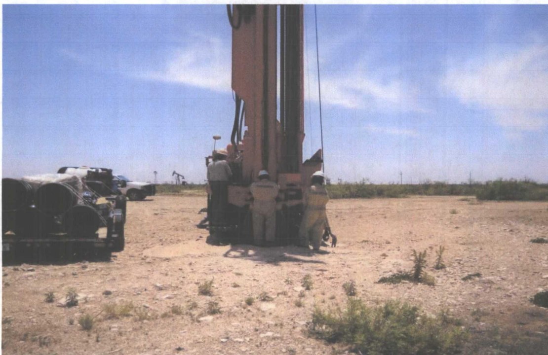
Chevron Grayburg 6-Inch Sec. 6 (Historical) - Advancement of Monitor Well MW-2
