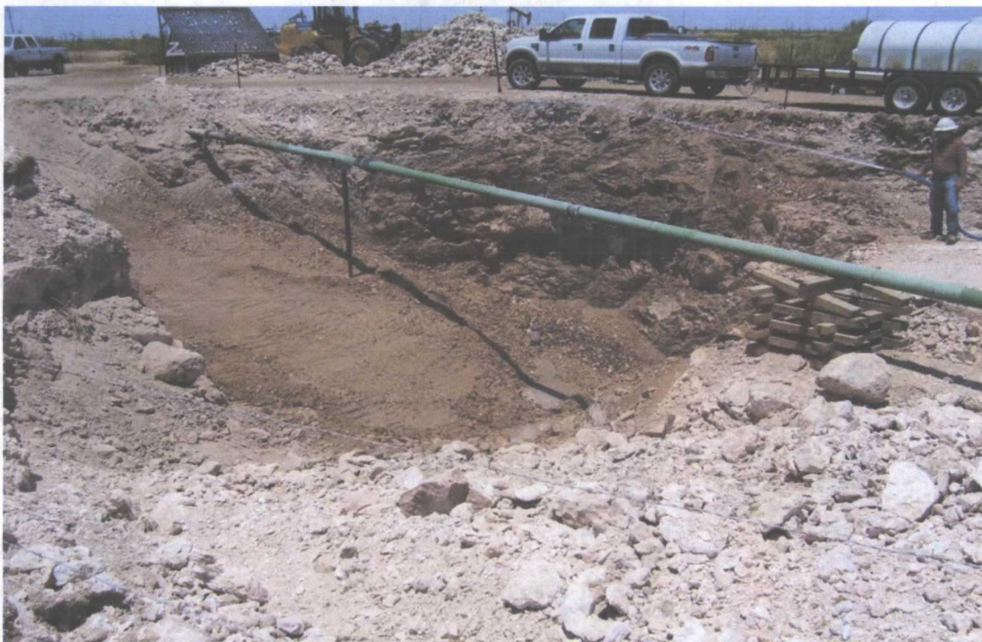
Chevron Grayburg 6-Inch Sec. 6 (Historical) - Excavation (Prior to Backfilling; Z-Screen & Screened Stockpile Visible in Background)
