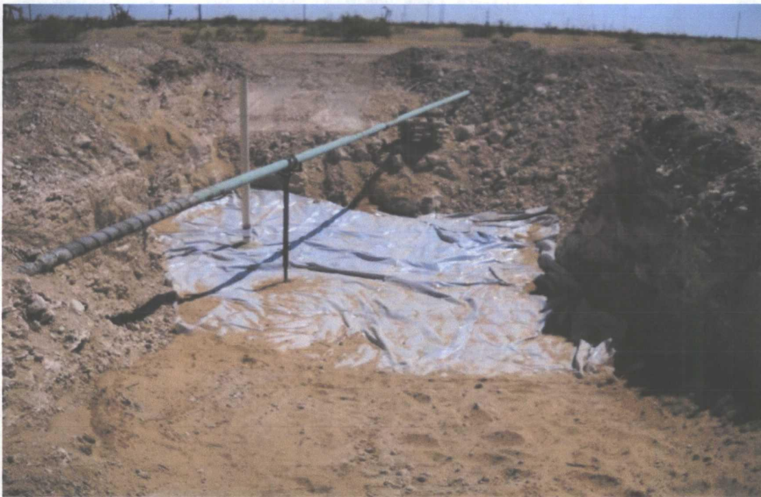
Chevron Grayburg 6-Inch Sec. 6 (Historical) - Excavation (Following Installation of 20-mil Liner & PVC Conduit)
