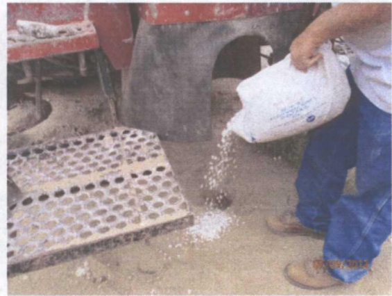
Plugging SB-1 in total with bentonite
