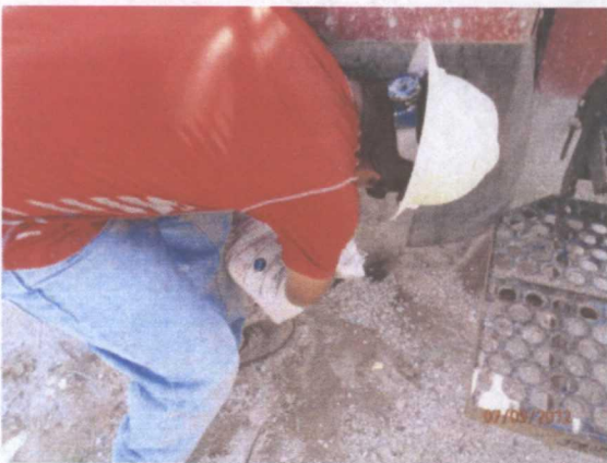
Plugging SB-4 in total with bentonite 7/9/12
