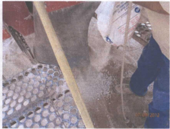
Plugging SB-5 in total with bentonite
