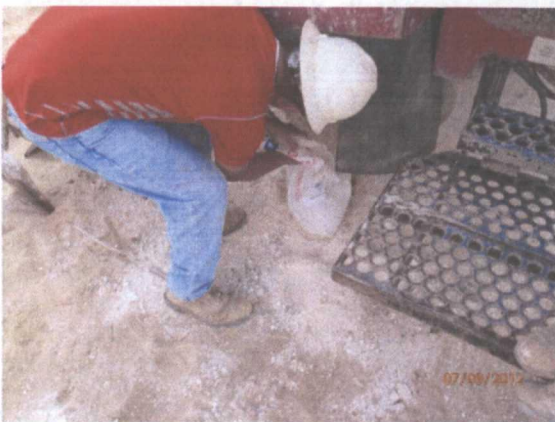
Plugging SB-2 in total with bentonite
