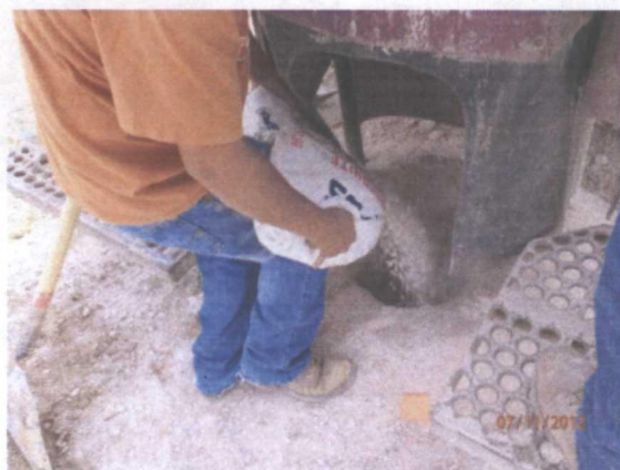
Plugging SB-2 in total with bentonite
