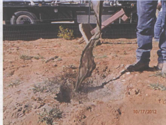
Plugging MW-1 with a 1-3% bentonite/concrete slurry and a 3 ft concrete cap
