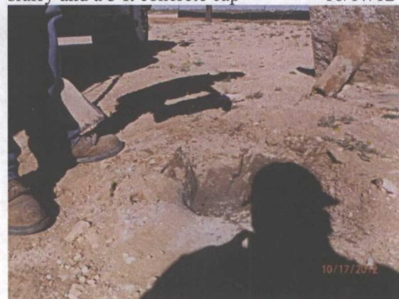
Plugging MW-3 with a 1-3% bentonite/concrete slurry and a 3 ft concrete cap
