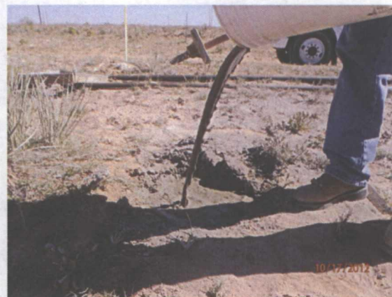
Plugging MW-2 with a 1-3% bentonite/concrete slurry and a 3 ft concrete cap
