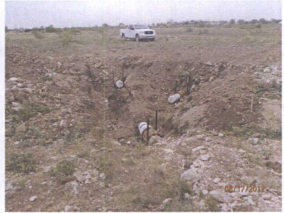
valves removed and pipe capped, facing NW 8/17/2012
