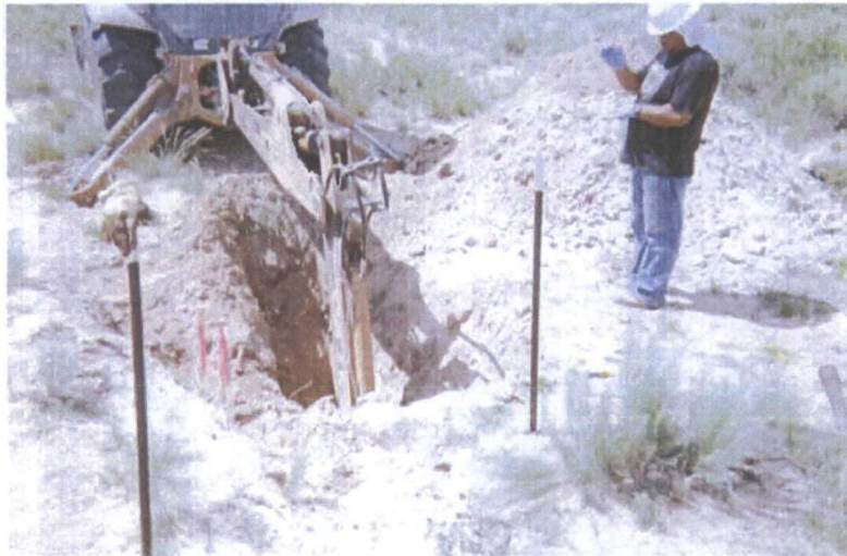
DELINEATION TRENCH BEING EXCAVATED
