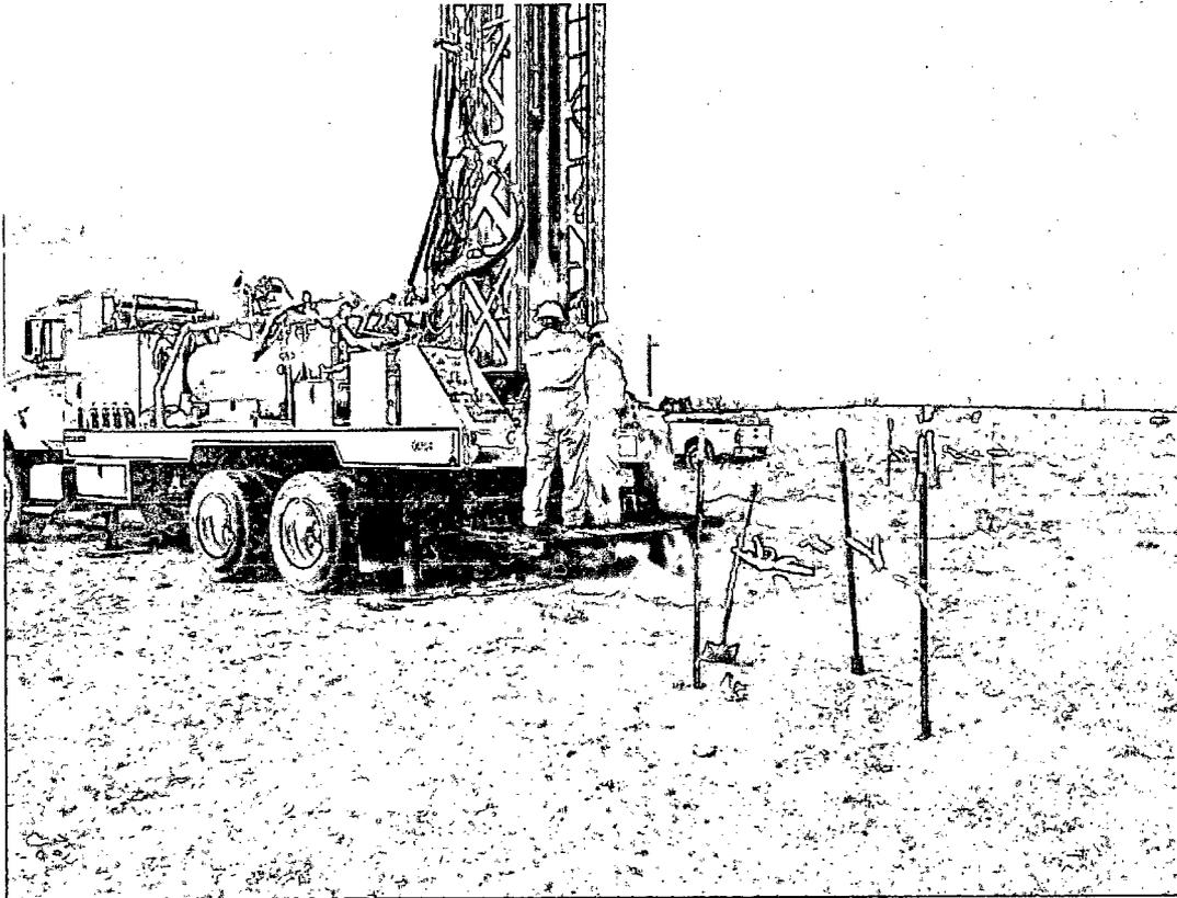
Photograph of advancement of soil bores and collection of core sample at the A-14 6" Line Historical Release Site.
