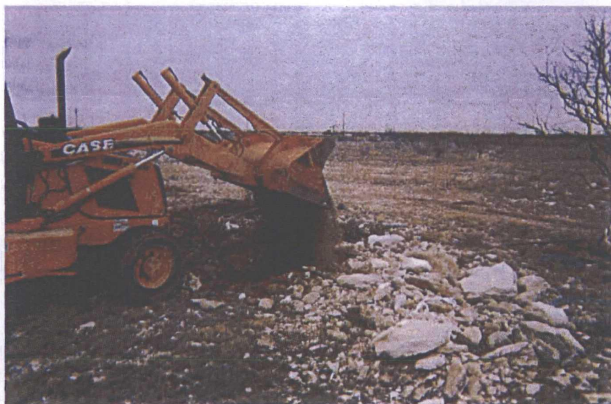
Backfilling excavation
