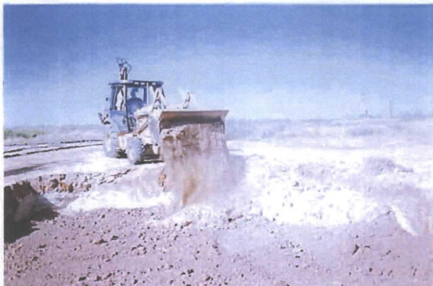
Backfilling excavation above clay liner
