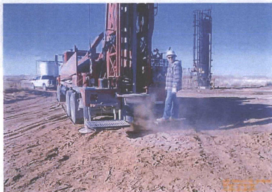
Installing Soil Bore
