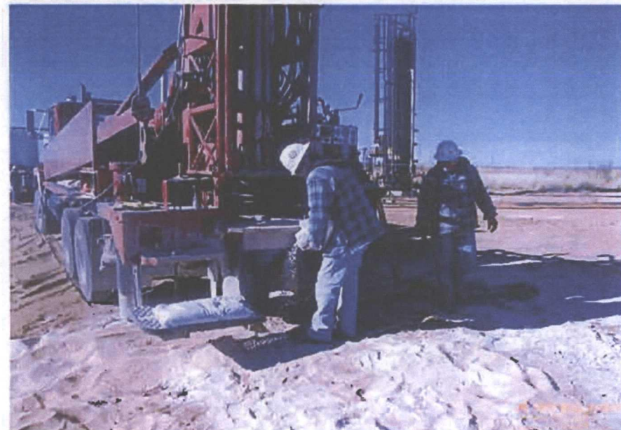
Plugging the soil bore with bentonite
